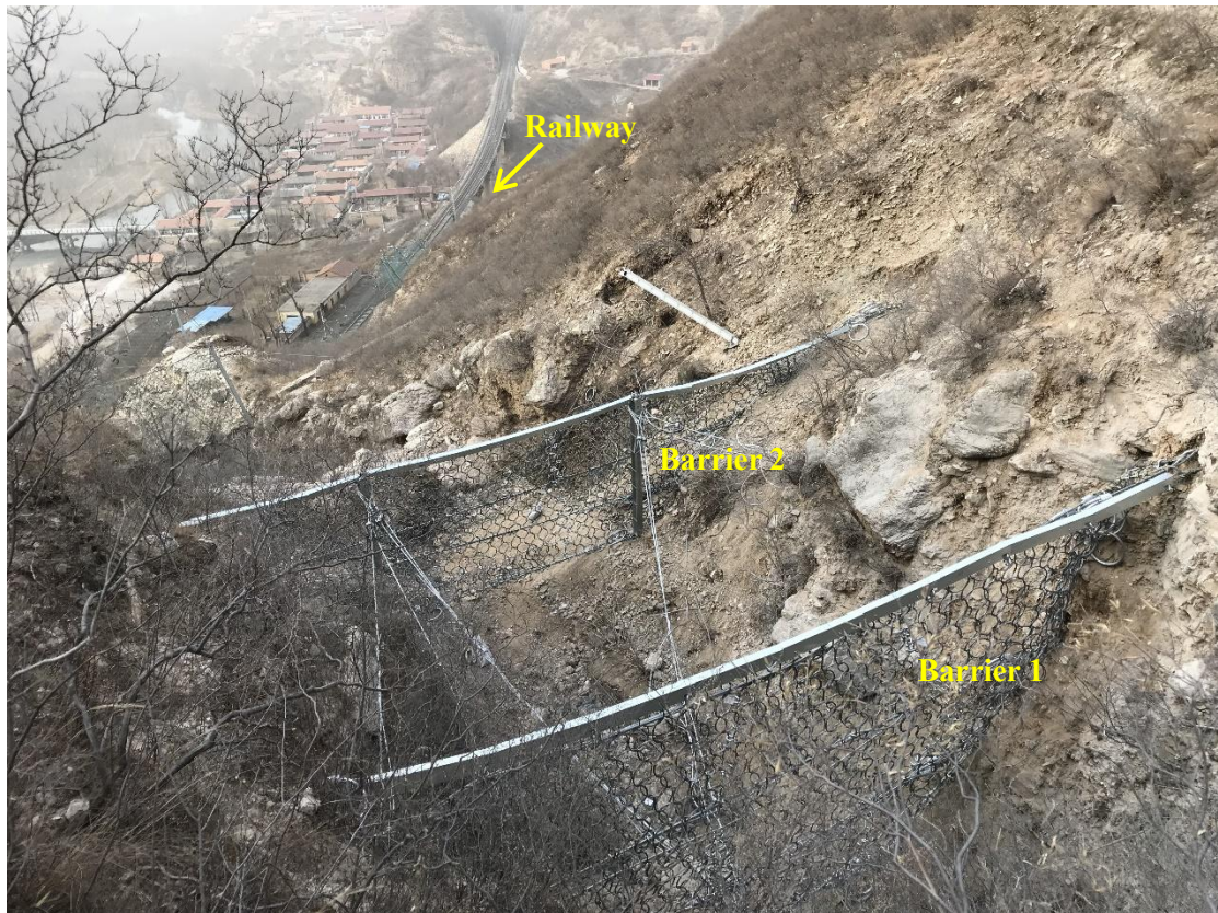
Fig. 1. Closely installed multiple debris-flow flexible barriers upstream a railway at west of Beijing.
