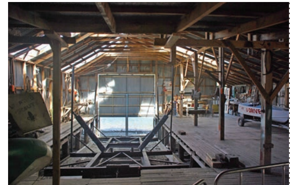
AFTER: THE LARGER SLIPWAY LOOKING FROM THE OPPOSING DIRECTION. THE SMALLER SLIPWAY IS ON THE LEFT AND HAS THE REMOVABLE FLOOR COVERING IN PLACE FOR WORKSPACE AND SAFETY REASONS.
