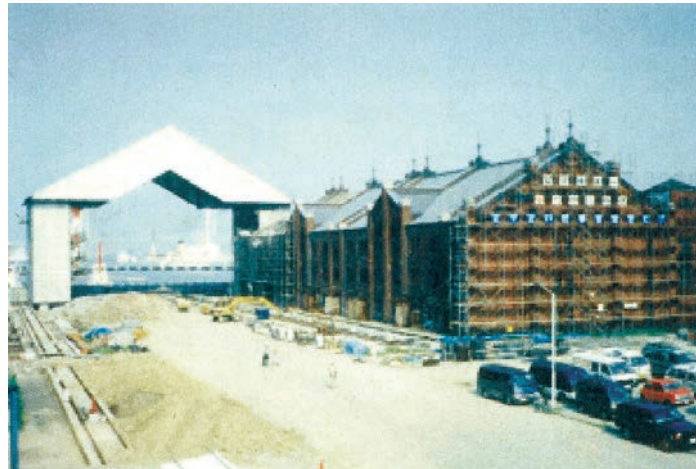
A TEMPORARY SLIDING ROOF WAS USED DURING THE CONSTRUCTION WORK
