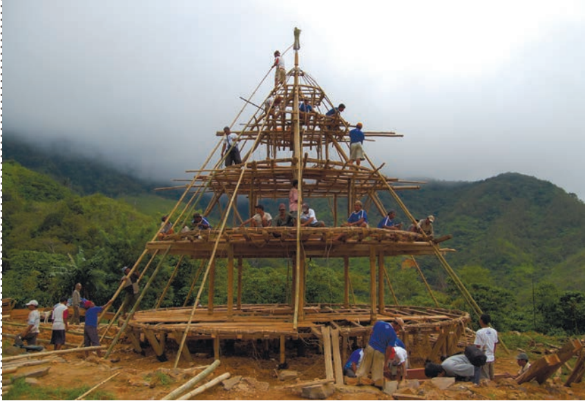
CONSTRUCTION OF THE TIRTA GENA JEKONG
