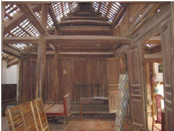
HA VAN VINH HOUSE TIMBER STRUCTURE
