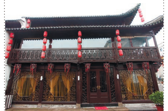
TEA HOUSE BEFORE AND AFTER CONSERVATION
