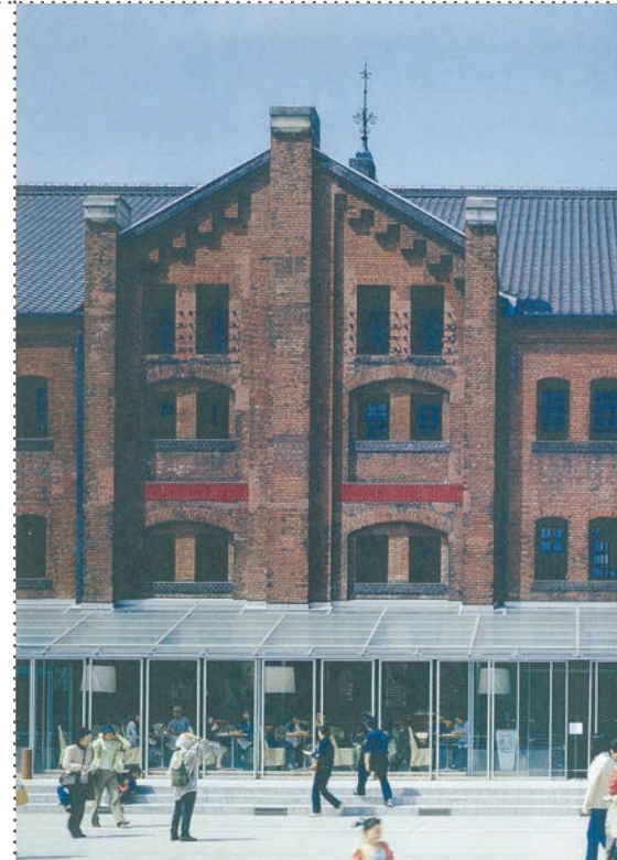
FRONT VIEW OF THE RESTORED BUILDING
