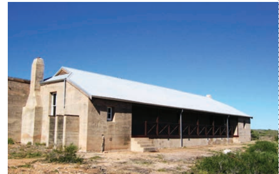
BEFORE AND AFTER RESTORATION
