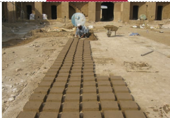
HANDMADE ADOBE BRICKS
