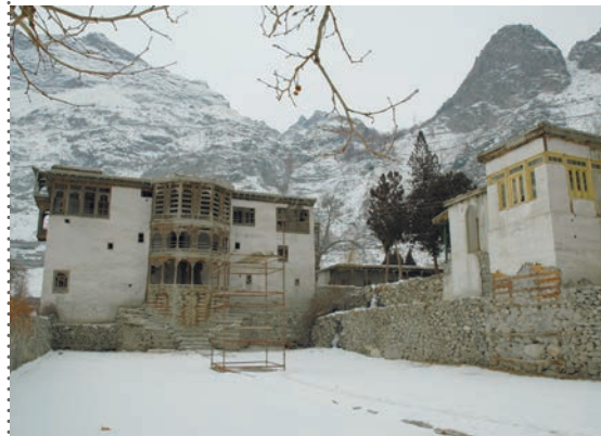
KHAPLU PALACE BEFORE RESTORATION
