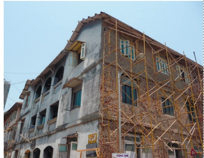
REPLACEMENT OF PLASTERWORK
