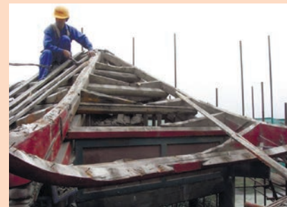
WORK IN PROGRESS ON THE HUAI'GU PAVILION ROOF
