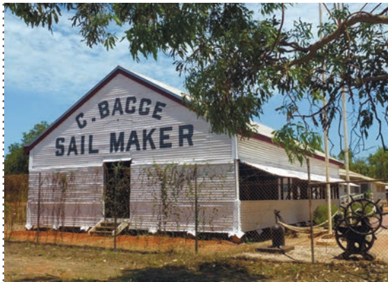
SAIL MAKER'S SHED BEFORE AND AFTER RESTORATION
