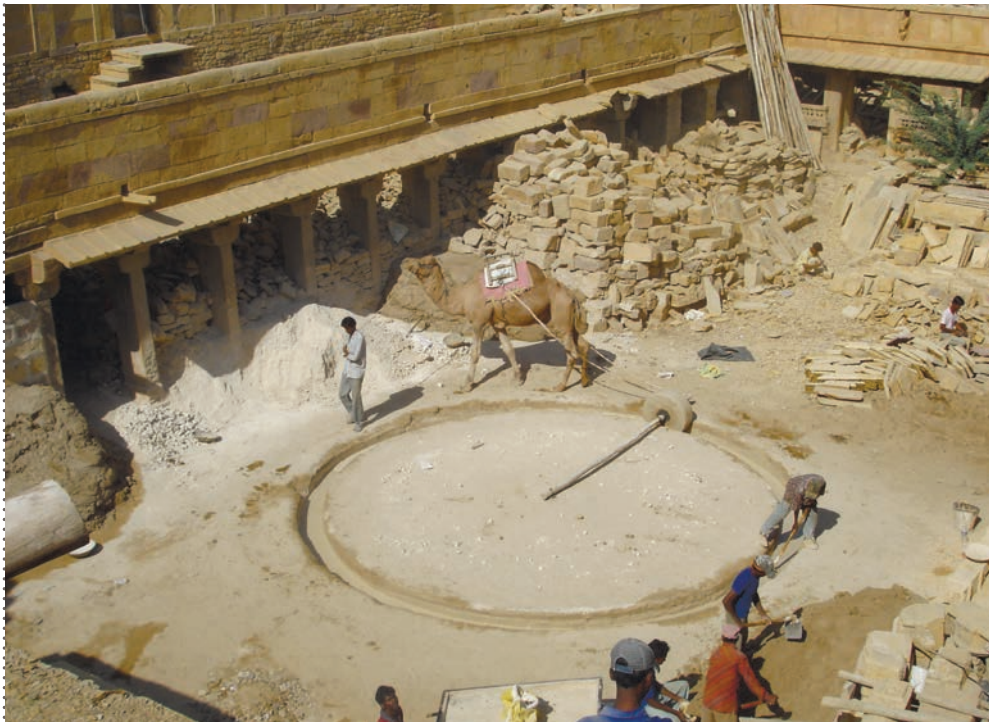
PRODUCING LIME MORTAR WITH TRADITIONAL LIME MILL
