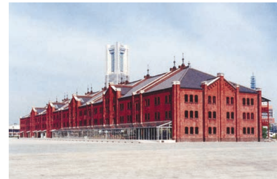
WAREHOUSE 2 AFTER RESTORATION, INCLUDING THE ADDED GLASS ANNEX
