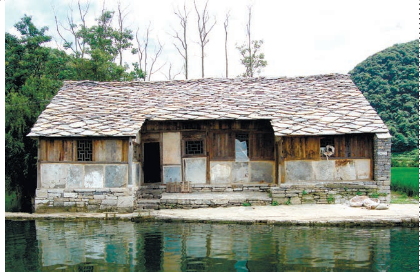
FRONT VIEW BEFORE AND AFTER RESTORATION
