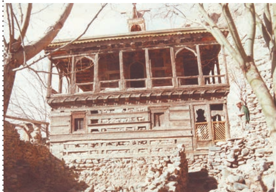
EXTERIOR BEFORE RESTORATION
