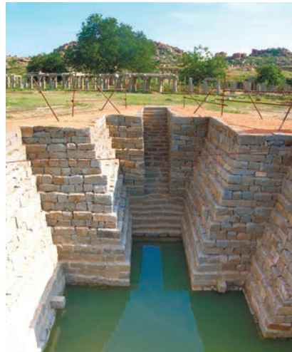
STEPPED WELL AFTER RESTORATION
