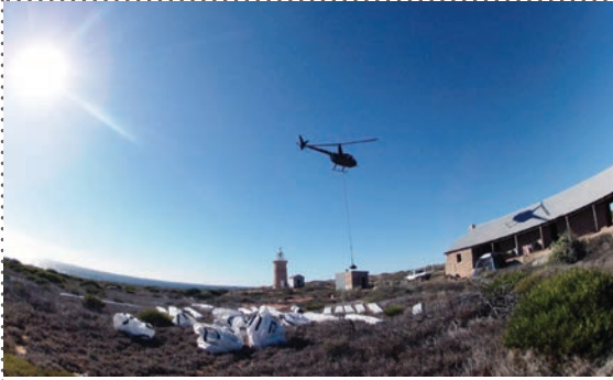
DELIVERY OF MATERIALS BY HELICOPTER.
