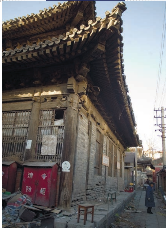
EXTERIOR BEFORE RESTORATION
