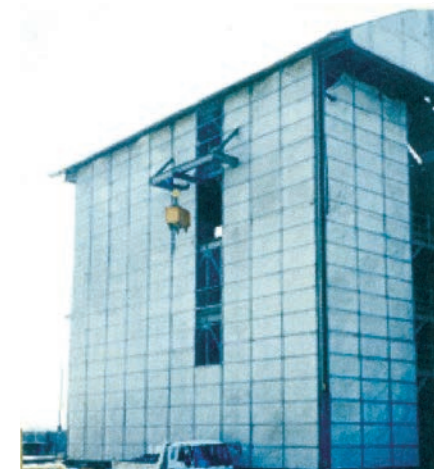
A TEMPORARY SLIDING ROOF WAS USED DURING THE CONSTRUCTION WORK
