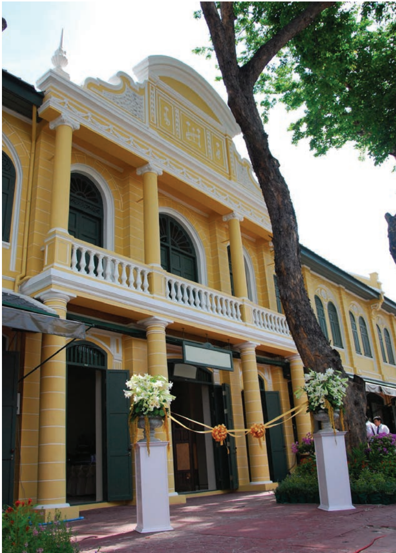
RESTORING THE NA PHRA LAN HISTORIC SHOPHOUSES CONTRIBUTED TO URBAN REVITALIZATION
