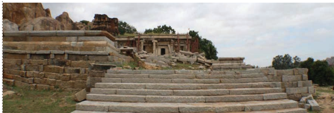
UPPER EMBANKMENT WALL BEFORE AND AFTER CONSERVATION
