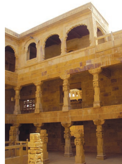
EXTERNAL WALL AFTER CONSERVATION
