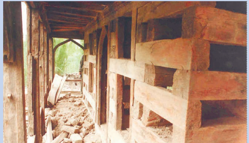
POPLAR WOOD IS USED ALONGSIDE STONE AND SOIL
