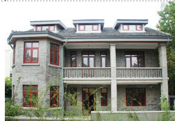
MANSION EXTERIOR BEFORE AND AFTER RESTORATION
