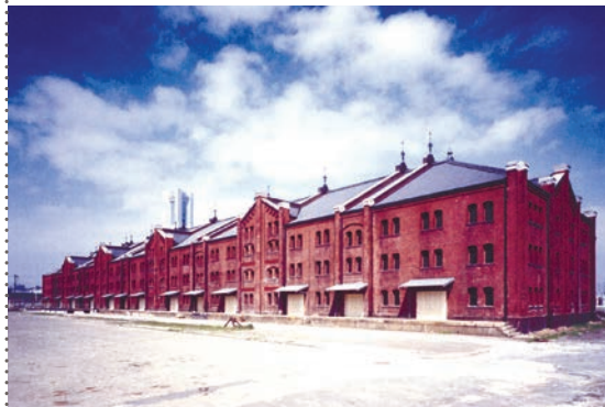
EXTERIOR OF WAREHOUSE 2 BEFORE RESTORATION
