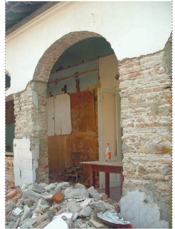
REDISCOVERED ARCHES DURING THE CONSERVATION WORKS
