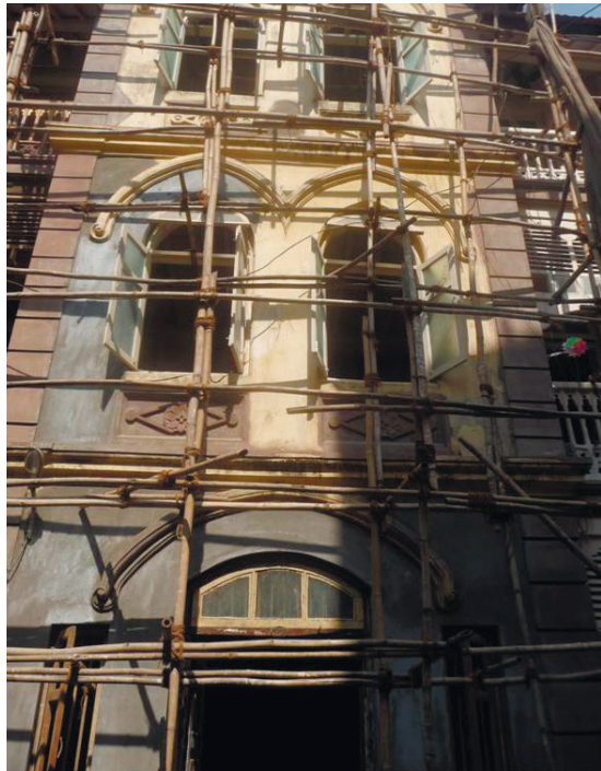
COOPER BUILDING BEFORE AND AFTER RESTORATION
