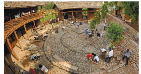
CONSTRUCTION OF THE COURTYARD
