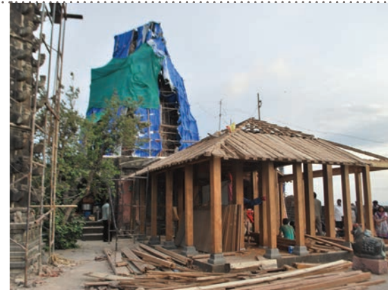
COMPLEX BEFORE AND DURING RESTORATION
