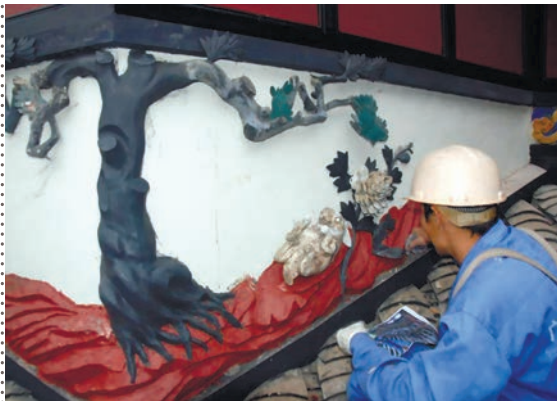
CONSERVATION WORK ON THE ROOF RIDGE DECORATIONS
