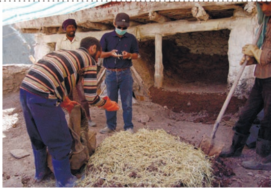
MIXING PHUGMA (WHEAT STRAW) WITH MUD FOR ROOFING
