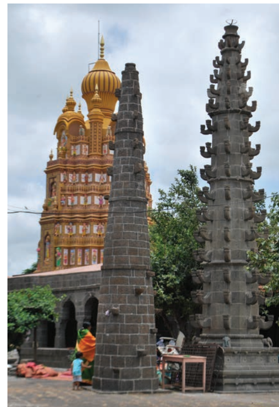
RESTORED SHIKHAR AND DEEPMALA
