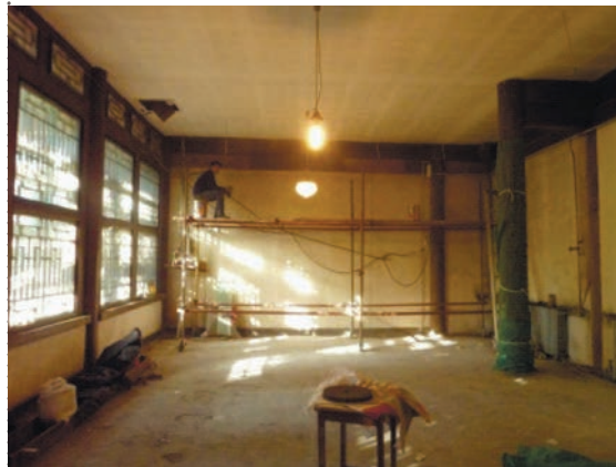
INTERIOR OF THE MAIN HALL BEFORE RENOVATION
