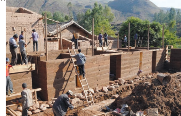
REINFORCING THE RAMMED EARTH BUILDINGS
