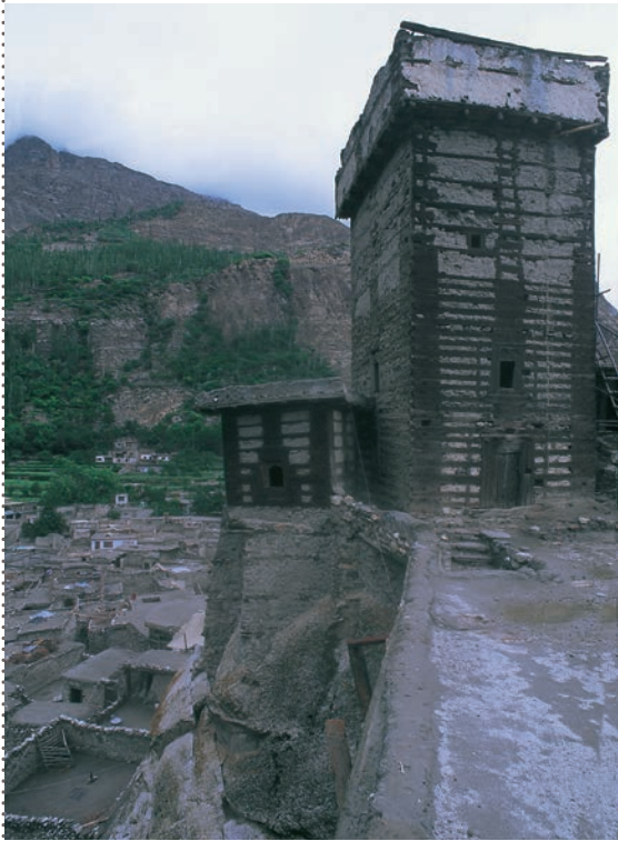
NORTH WEST ELEVATION BEFORE RESTORATION
