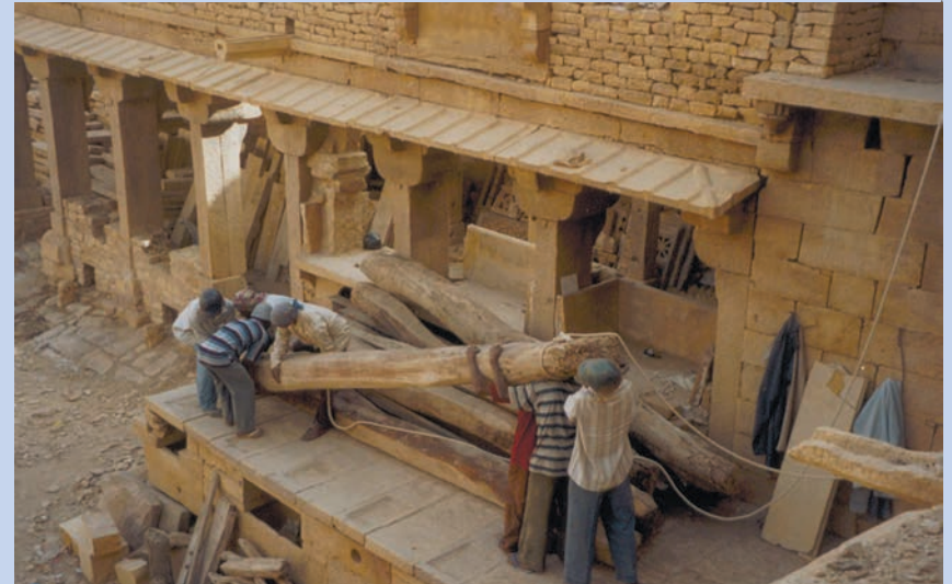
MOVING BEAMS INTO PLACE
