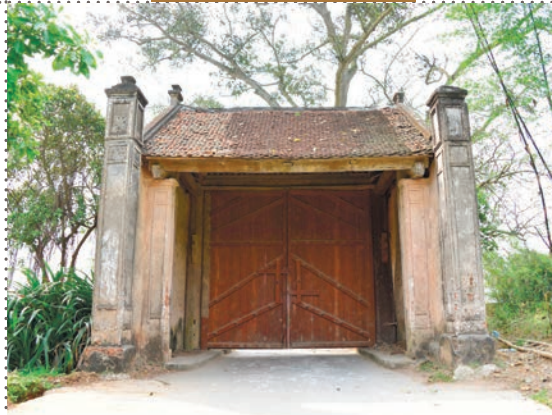
MONG PHU GATE AFTER RESTORATION
