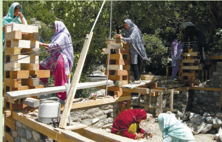
CIQAM MEMBERS DOING CARPENTRY WORK
