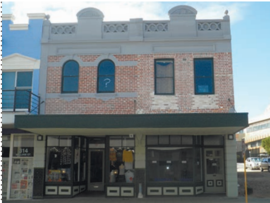
HISTORIC FAÇADE DETAILS HAVE BEEN REVEALED
