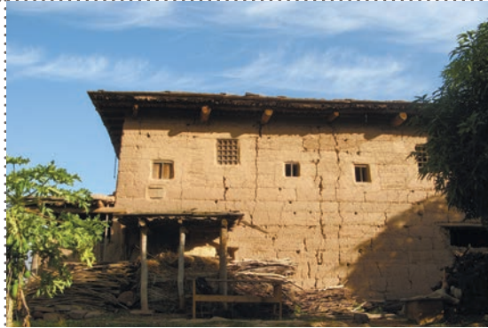
THE PROTOTYPE HOUSE BEFORE RECONSTRUCTION
