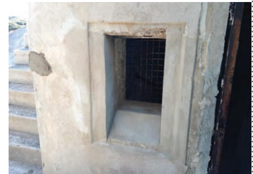
BICKLEY BATTERY WINDOWS BEFORE AND AFTER RESTORATION
