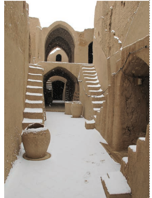
INTERIOR PASSAGE BEFORE AND AFTER RESTORATION
