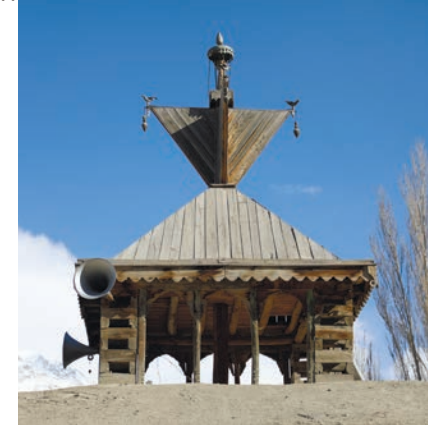
TOWER AFTER RESTORATION
