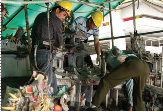
COMPONENTS ON THE ROOF BEING REMOVED FOR CONSERVATION TREATMENT
