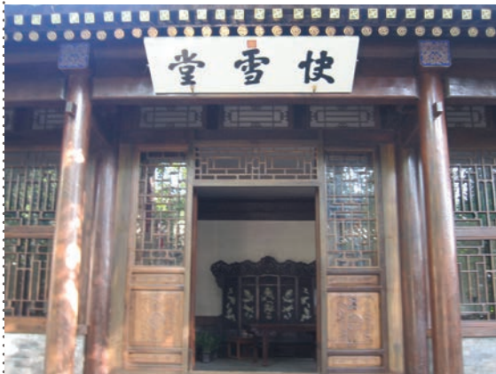
ENTRANCE TO THE ENJOYING SNOW HALL (MAIN HALL) AFTER RENOVATION
