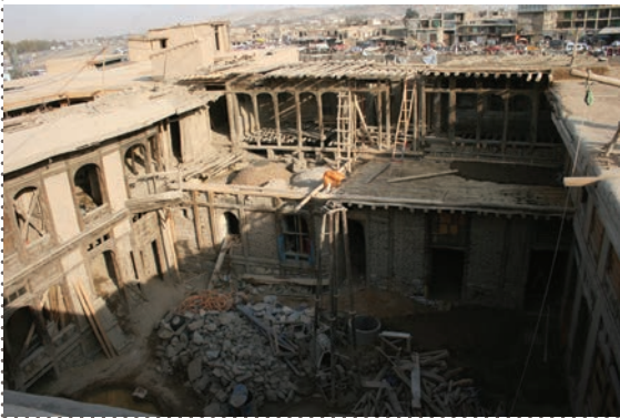
EXTERIOR OF THE GREAT SERAI BEFORE RESTORATION
