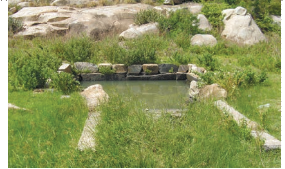
STEPPED WELL BEFORE CONSERVATION
