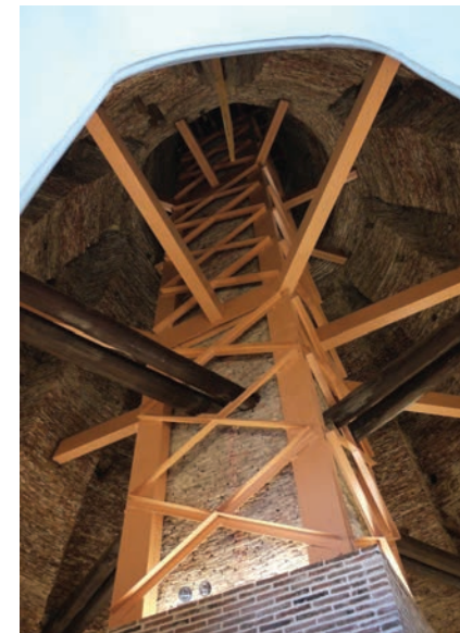
THE LEANING CENTRAL PILLAR (LEFT) WAS STRAIGHTENED AND BRACED (RIGHT)
