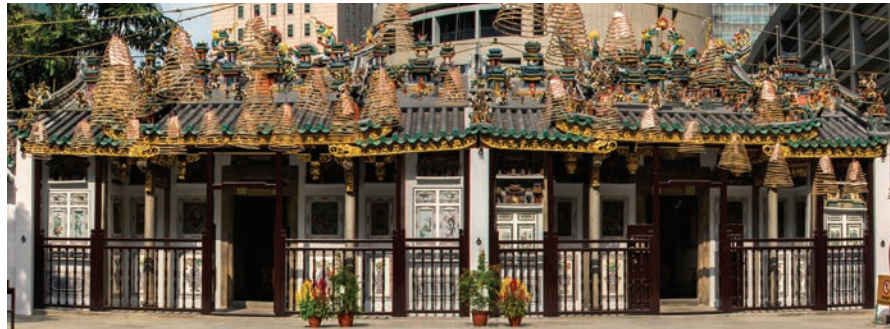
FRONT ELEVATION OF TEMPLE AFTER CONSERVATION
