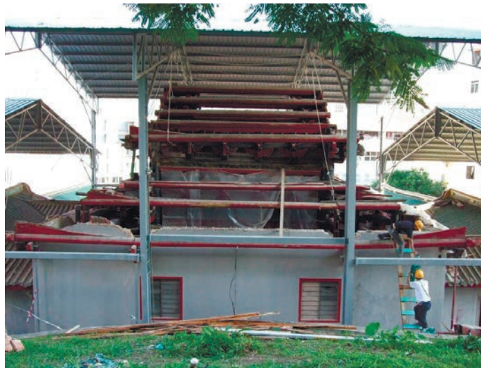
TEMPORARY DISMANTLING OF THE MAIN HALL ROOF
