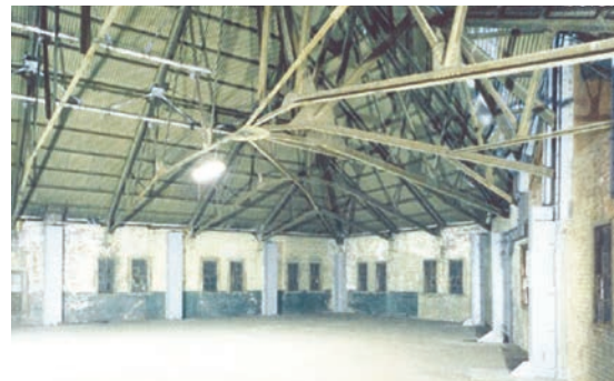
INTERIOR OF WAREHOUSE 2 BEFORE RESTORATION
