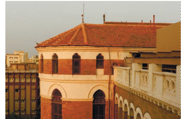
REPAIRS TO THE ROOF (DURING AND AFTER)
