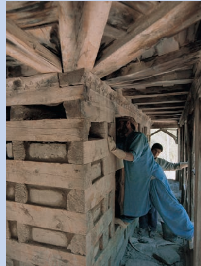
TIMBER FRAMED STRUCTURE
