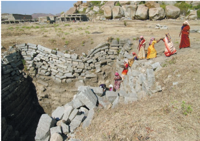
LOCAL WORKERS REBUILDING STEPPED WELL
