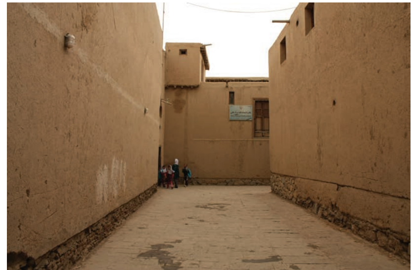
URBAN SERVICES WERE UPGRADED AROUND THE GREAT SERAI
