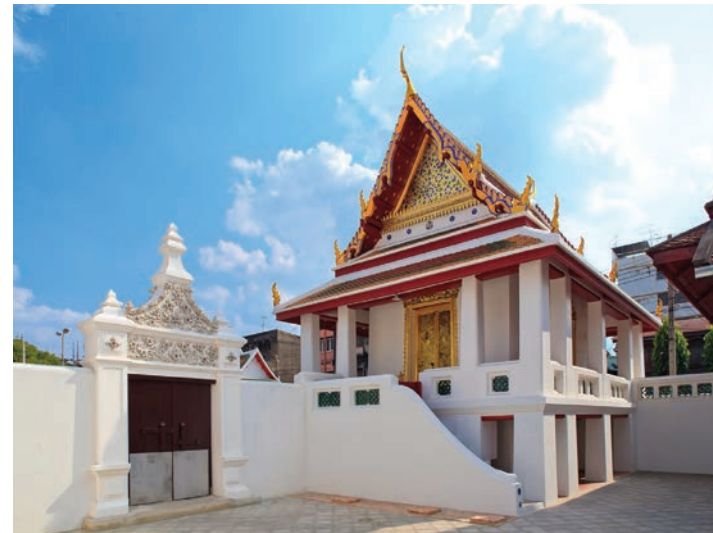
EXTERIOR BEFORE AND AFTER RESTORATION
