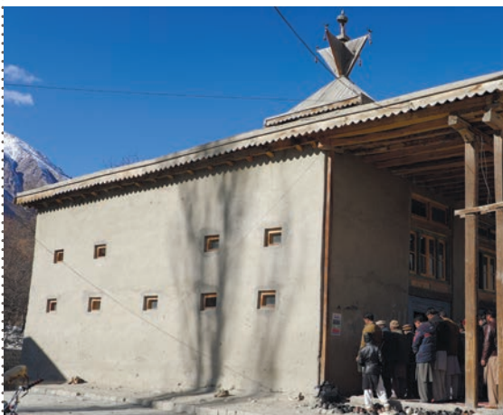
SOUTH ELEVATION BEFORE, DURING AND AFTER RESTORATION
