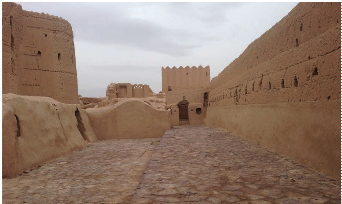
INTERIOR COURTYARD AFTER RESTORATION
