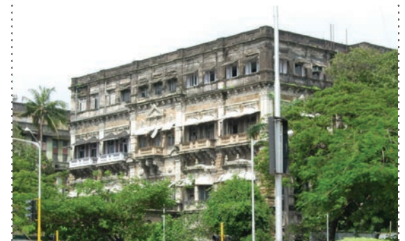
FAÇADE BEFORE AND AFTER RESTORATION
