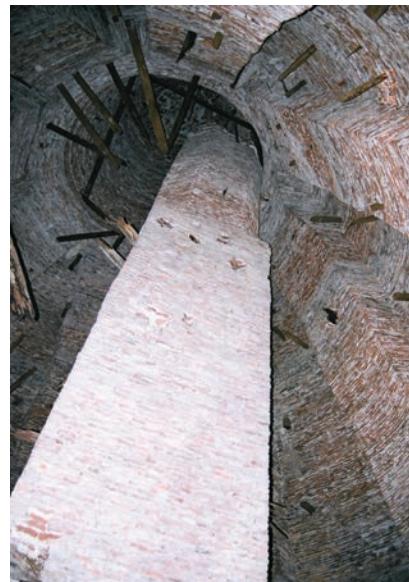
THE LEANING CENTRAL PILLAR (LEFT) WAS STRAIGHTENED AND BRACED (RIGHT)
