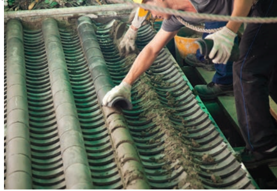
MOCK-UP ROOF TILING
