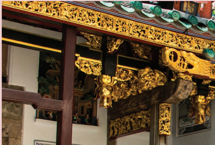
WOODEN ELEMENTS WERE INVESTIGATED
