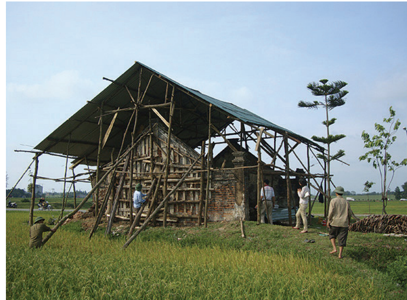
RESTORATION PROCESS OF A HISTORIC BUILDING IN DUONG LAM VILLAGE
