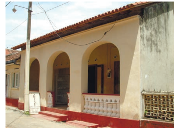
ONE OF THE PROJECT HOUSES BEFORE CONSERVATION
