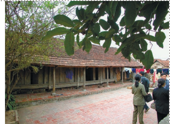
NGUYEN VAN HUNG HOUSE BEFORE RESTORATION
