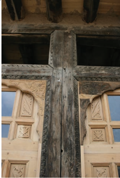
GLAZING INSERTS TO IMPROVE THE THERMAL PERFORMANCE OF PATAYI WERE MADE REVERSIBLE
