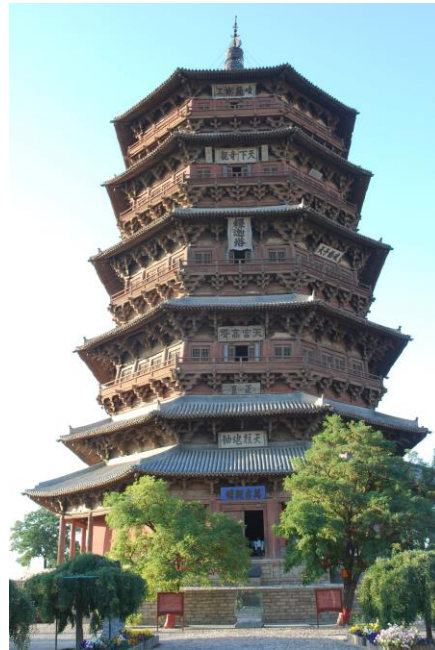
Fig. 1. The Yingxian timber pagoda, Shanxi Province, China [25]
