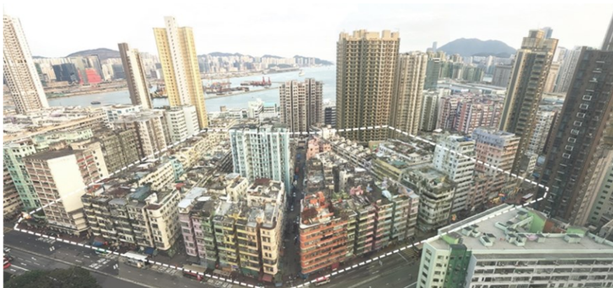
Figure 1. Existing condition of the To Kwa Wan site in Hong Kong
