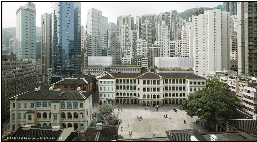
Figure 1: (Source: Commissioner for Heritage’s Office of the Development Bureau)
