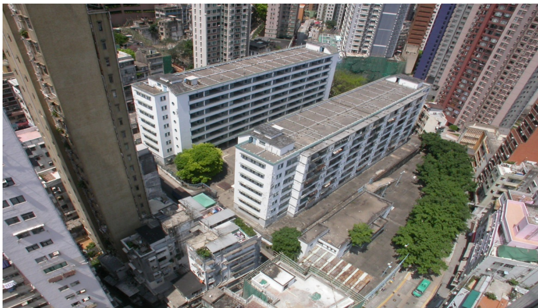
Figure 2 (Source: Commissioner for Heritage’s Office of the Development Bureau)
