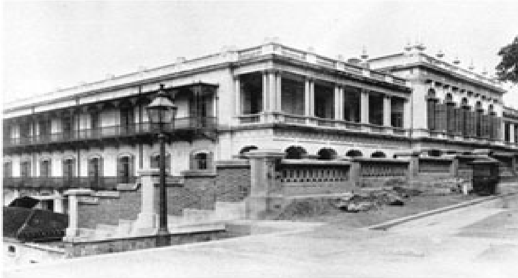
Figure 3 (Source: Commissioner for Heritage’s Office of the Development Bureau)
