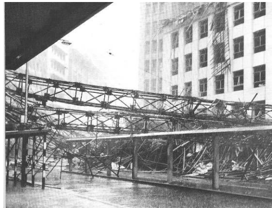
Figure 2a & b. Scaffolding damages Typhoon Wanda 1962, and Ruby 1964
