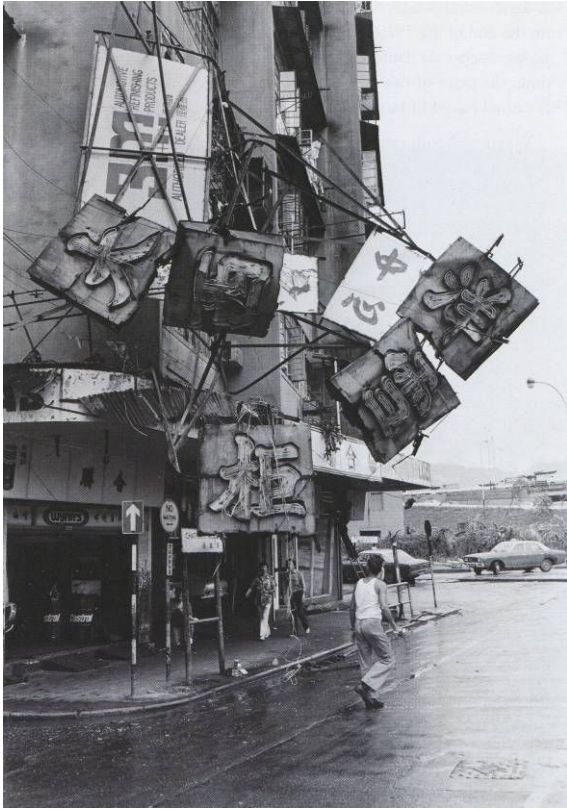
Figure 3a & b. Damages to sign boards Typhoon Hope 1979 and Wanda 1962
