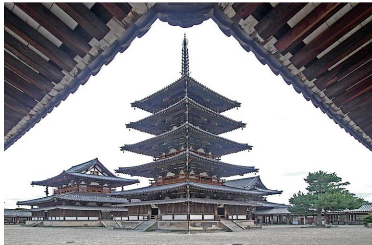
Figure 2. Five-Storied Pagoda at Horyuji, Nara
