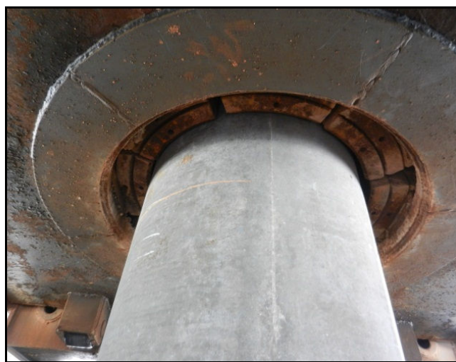
Figure 3: Clamping of PHC pile
