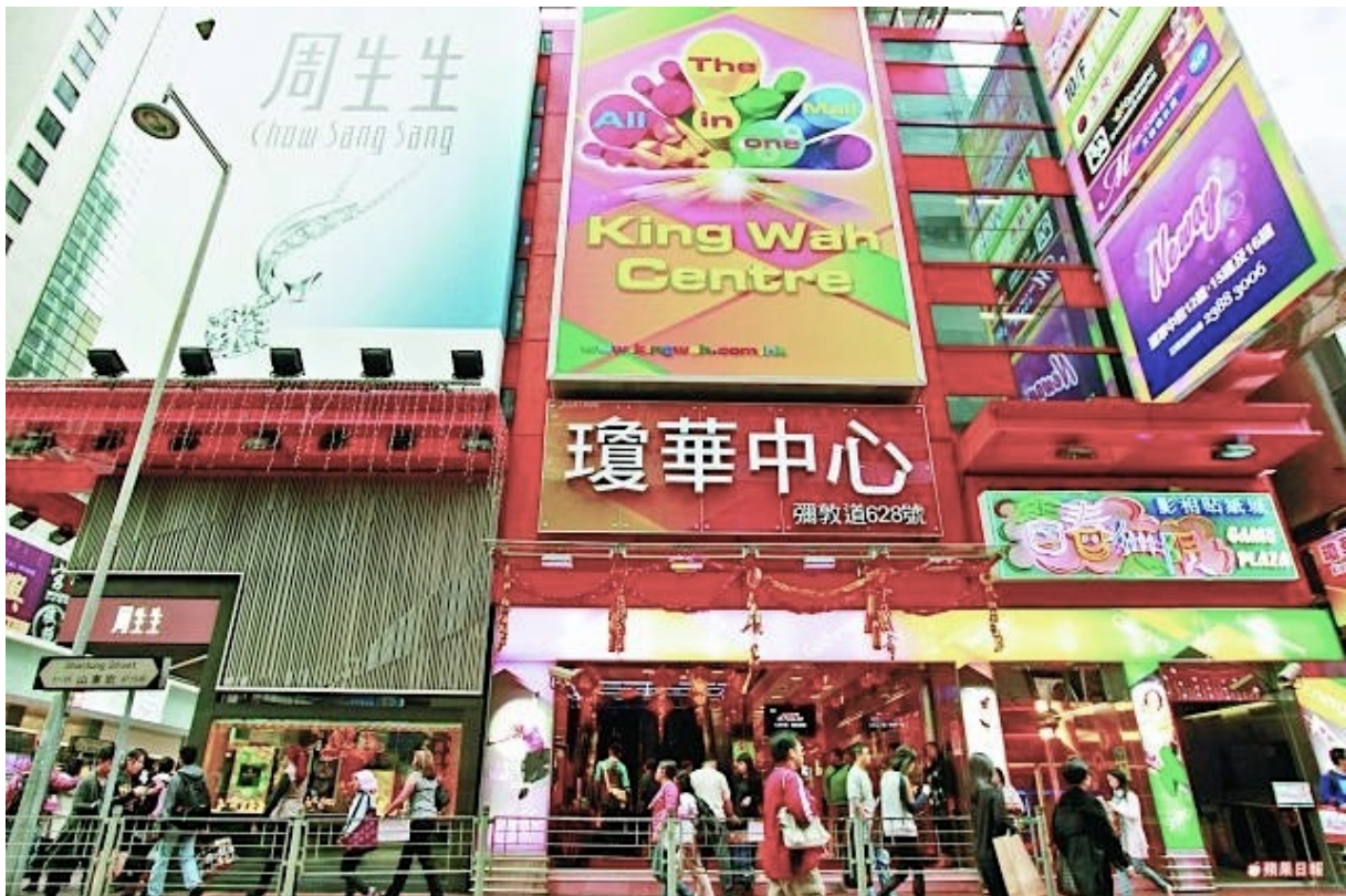
FIG. 1 King Wah Centre, one of the many older shopping malls in Hong Kong that is about to be demolished to make way for a more upscale shopping center, 2013. (Source: Apple Daily )
