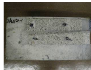
(c) Anchor rupture
