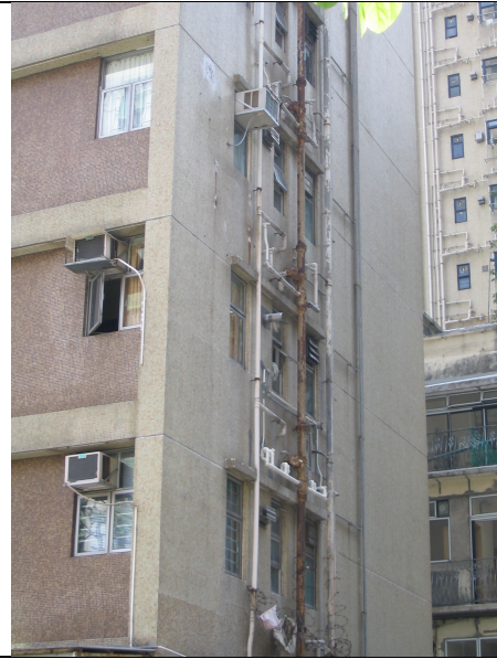
Close up view of low-grade exterior
