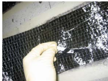
(b) Passing parted sheet fibres over FRP anchor
