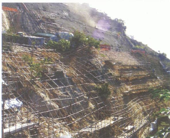
*Landslip prevention with soil nails and Drilling Process Monitor (DPM)*
