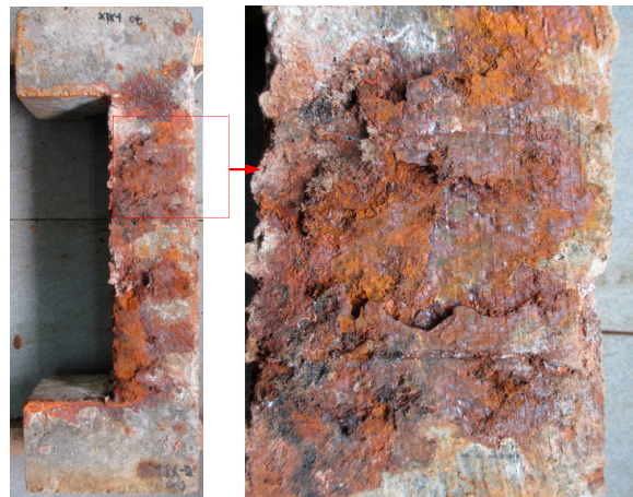
Figure 15. The damage in the RC column specimen caused by corrosion of the reinforcement.
